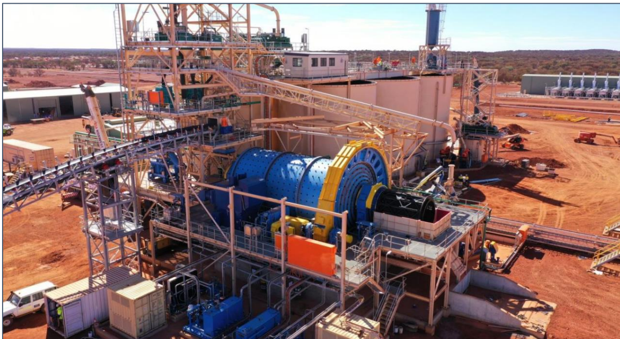
Ball mill installed and commissioning underway
